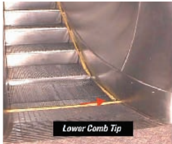
Bottom landing: Lower Comb Tip
