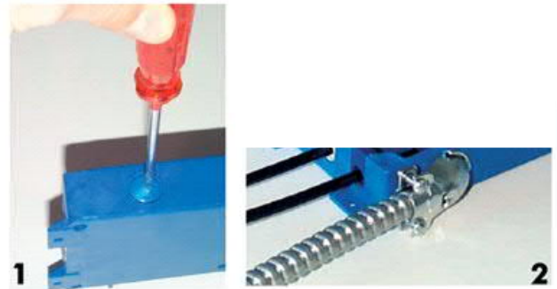
Figure 4: Installation of a Greenfield fitting
